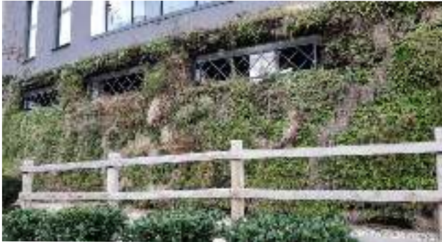
Figure 3: example of a green wall in an urban setting
