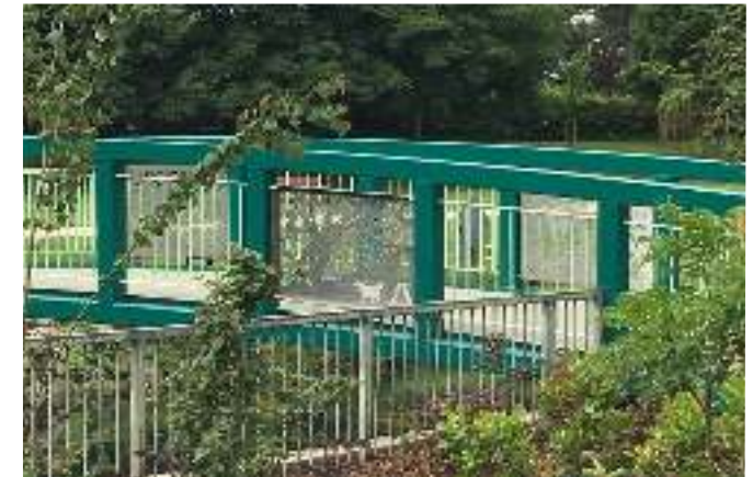
Figure 17: Green spaces interacting with the rivers and providing suitable river crossings to connect spaces
