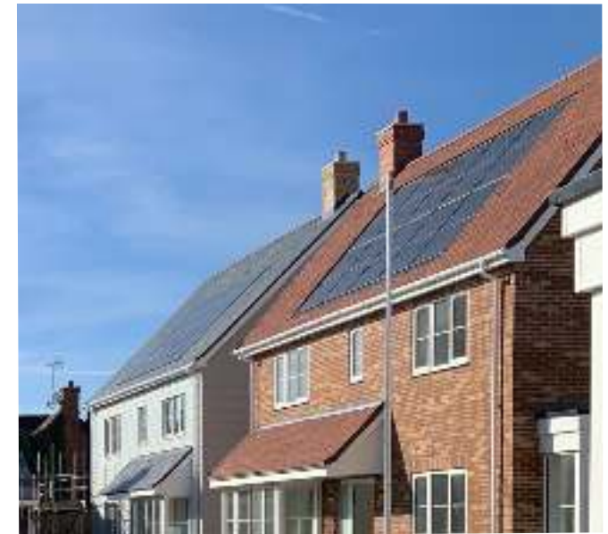
Figure 37: Integrated domestic solar panels
