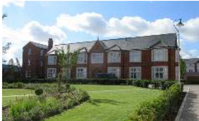
Figure 33: Conversion of a retained building within the conservation area at the St John's Hospital site, Chelmsford
