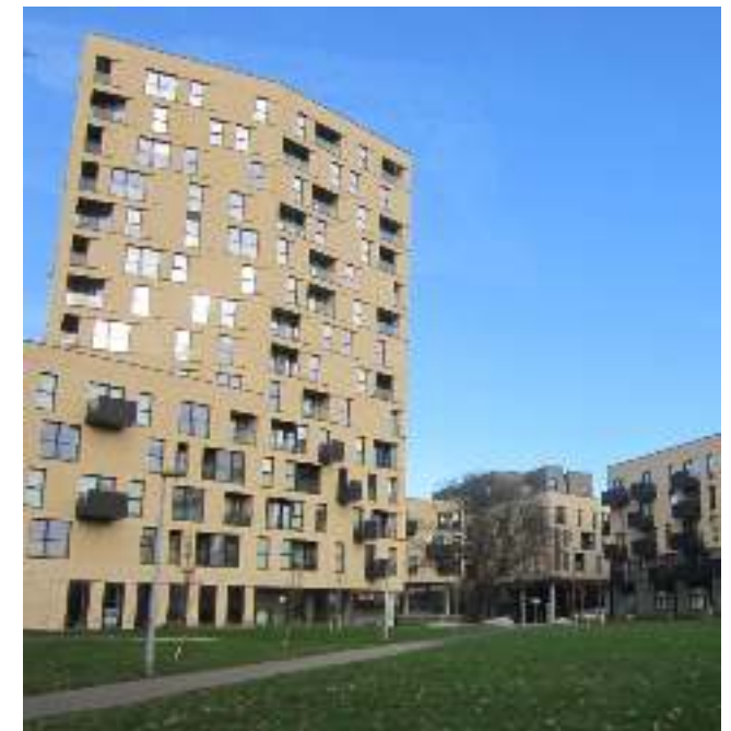
Figure 31: Tall buildings within City Park West development
