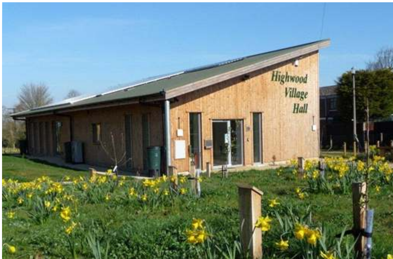
Figure 38: Highwood Village Hall is built to Passivhaus principles with excellent thermal performance and airtightness. The triple glazed windows are oriented to the south, west and east to maximise natural solar gain and the roof overhang provides shading. Solar panels and an air source heat pump provide electricity and heating.
