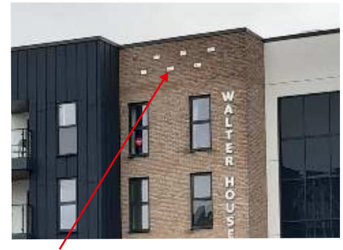
Figure 1: Swift bricks should be installed high up in gable ends or directly under eaves
