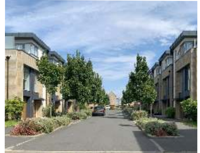
Figure 4: Trees reinforcing linear features, planting screening walls and shrubs between the road and the footway being part of the overall SUDS strategy.
