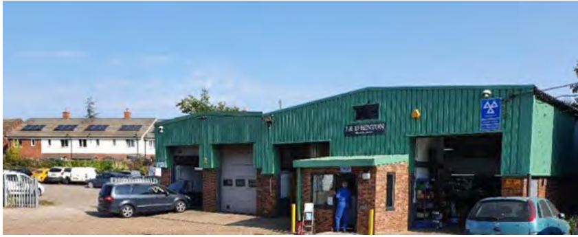
Commercial Unit at the Danbury Business Park.
