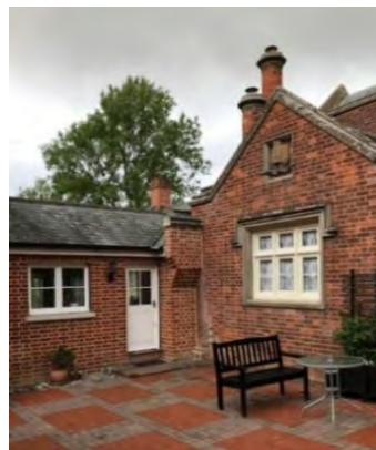
Before and after pictures of a single storey brick extension to a listed property.
