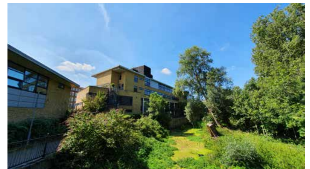
South east campus buildings adjacent to the River Chelmer
