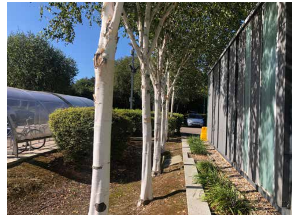
Example of existing swale (adjacent to Mildmay)
