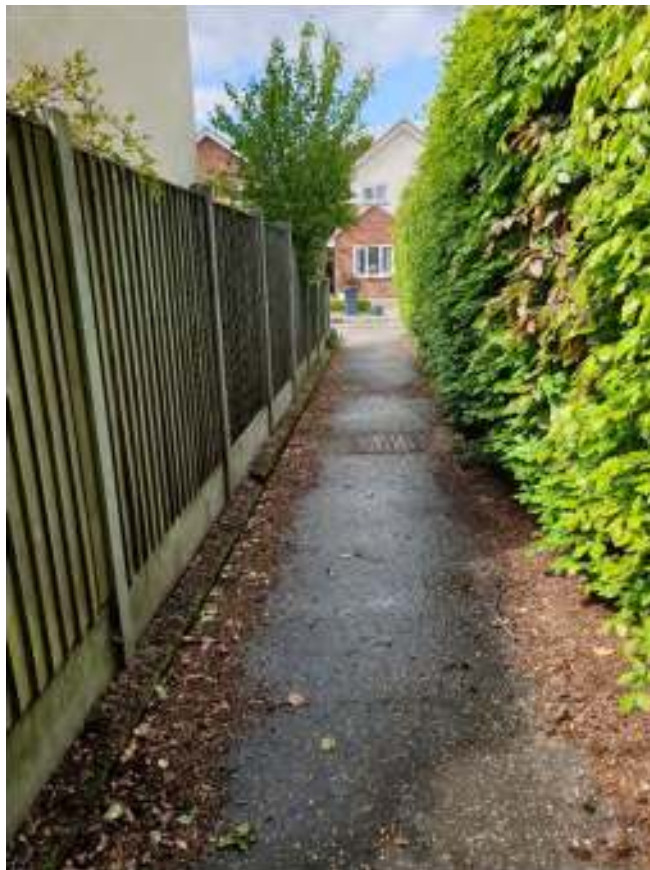
Image 2.7 - Existing Footway Surface – PROW Link
