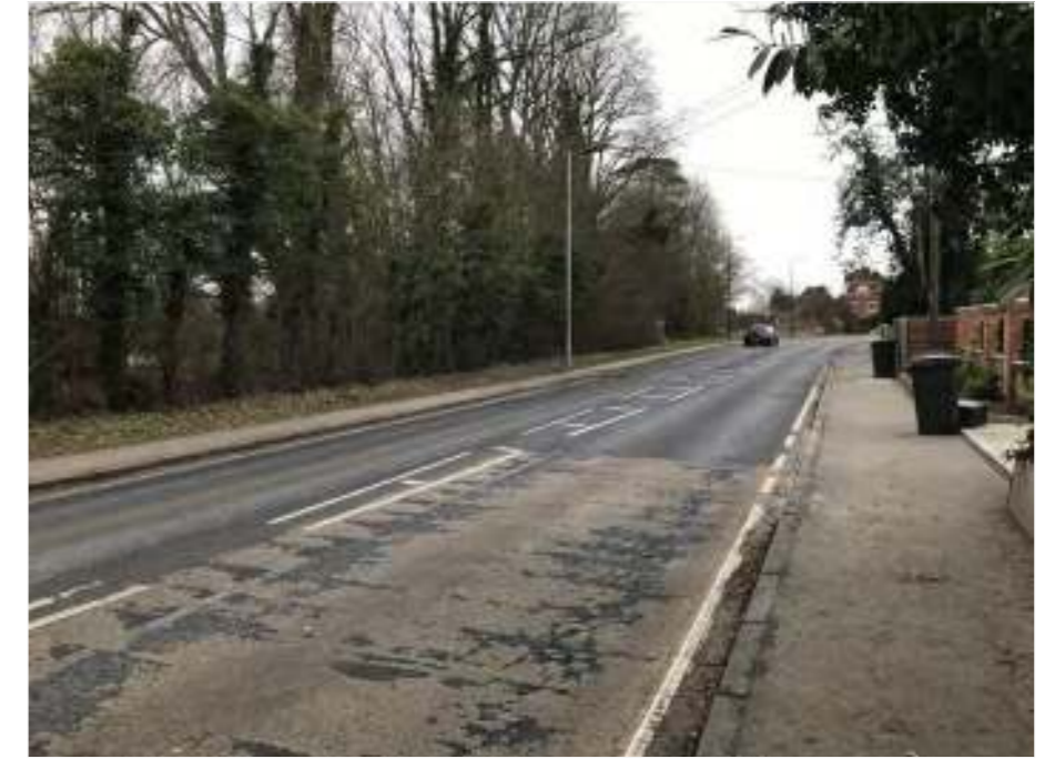
Figure 26: View towards Site from north-east of Maldon Road
