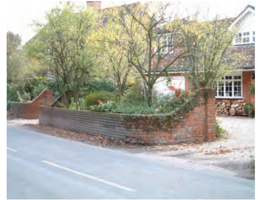
Low brick boundary wall in School Road
