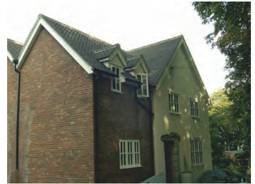
Extension using dormer windows
