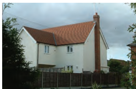
Plain tile roof and rendering at Farrier Square
