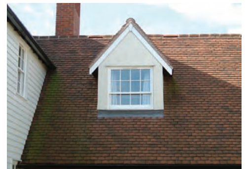
Pitched plain tile roof with dormer window
