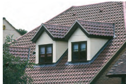
Roof conversion, Church Road
