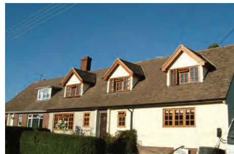
Roof conversion, Park Lane
