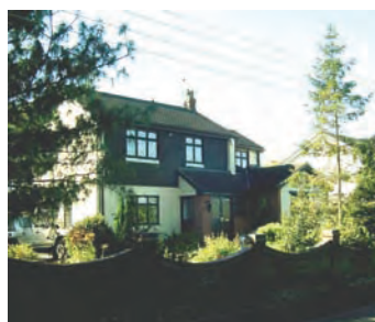
Bow top brick boundary wall
