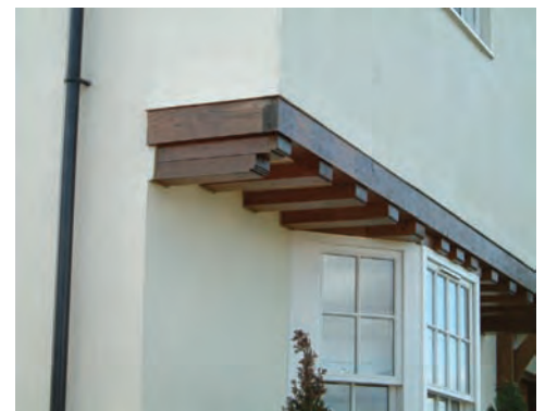
Cantilever floor detail
