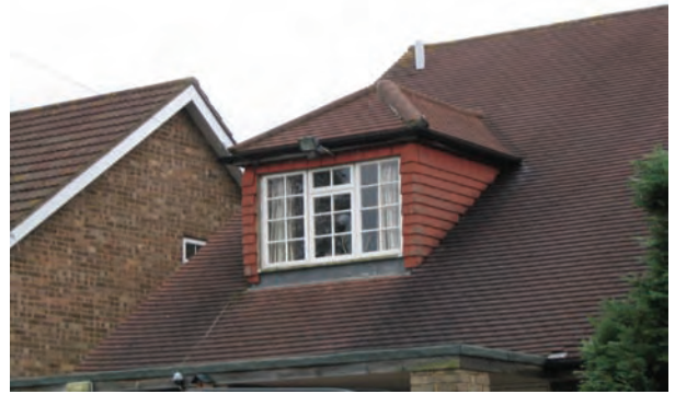
Dormer conversion Downham Road
