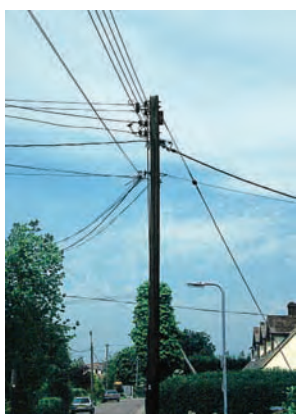
Overhead power lines
