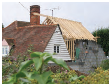
Extension in progress on cottage in Downham Road
