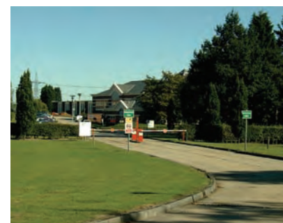
Hanningfield water treatment centre
