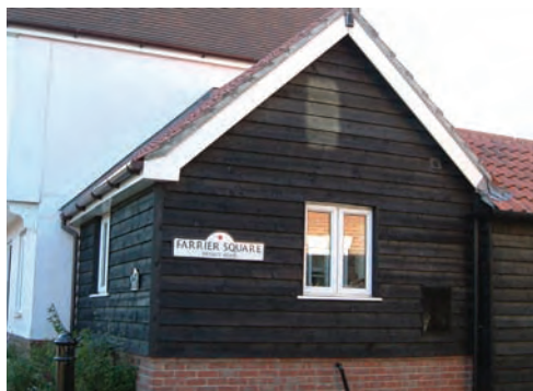
Weatherboarding at Farrier Square
